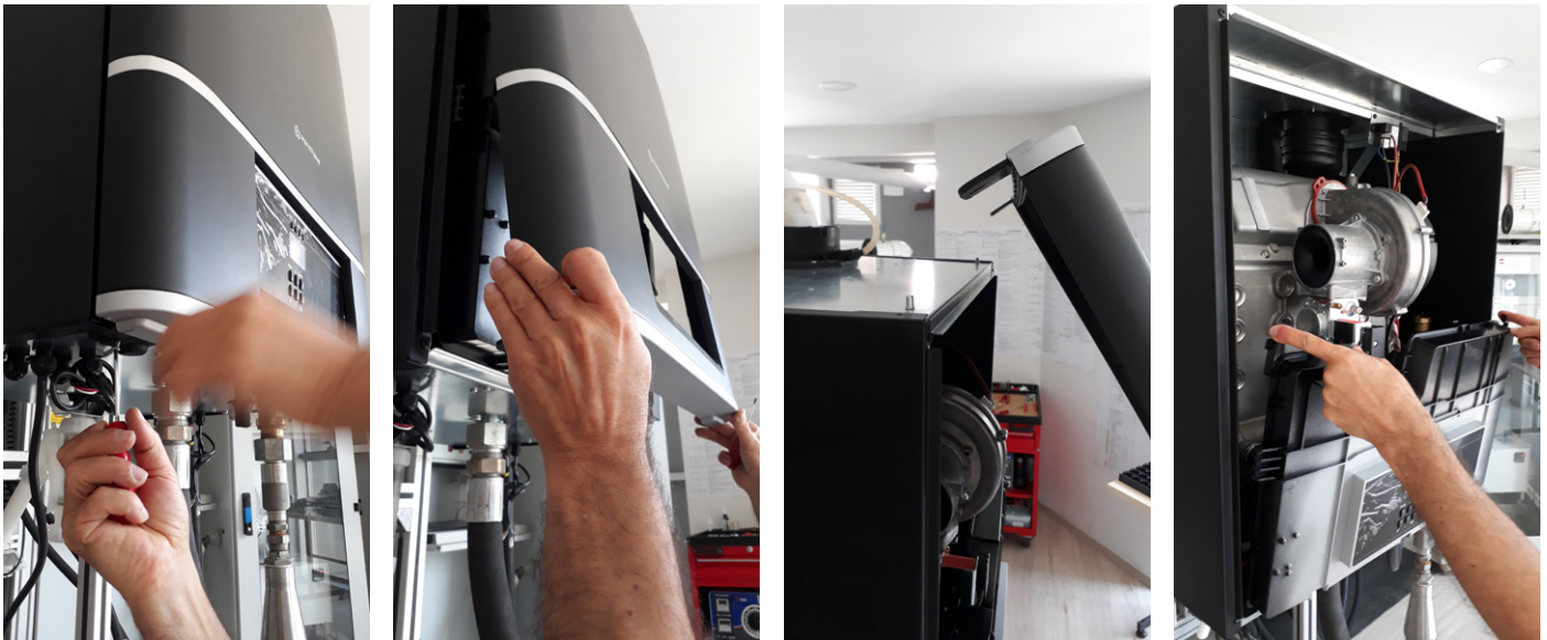
Figure 5.1 You can see the operation sequence for removing the front cover of boiler and controlling the connections of other parts.
